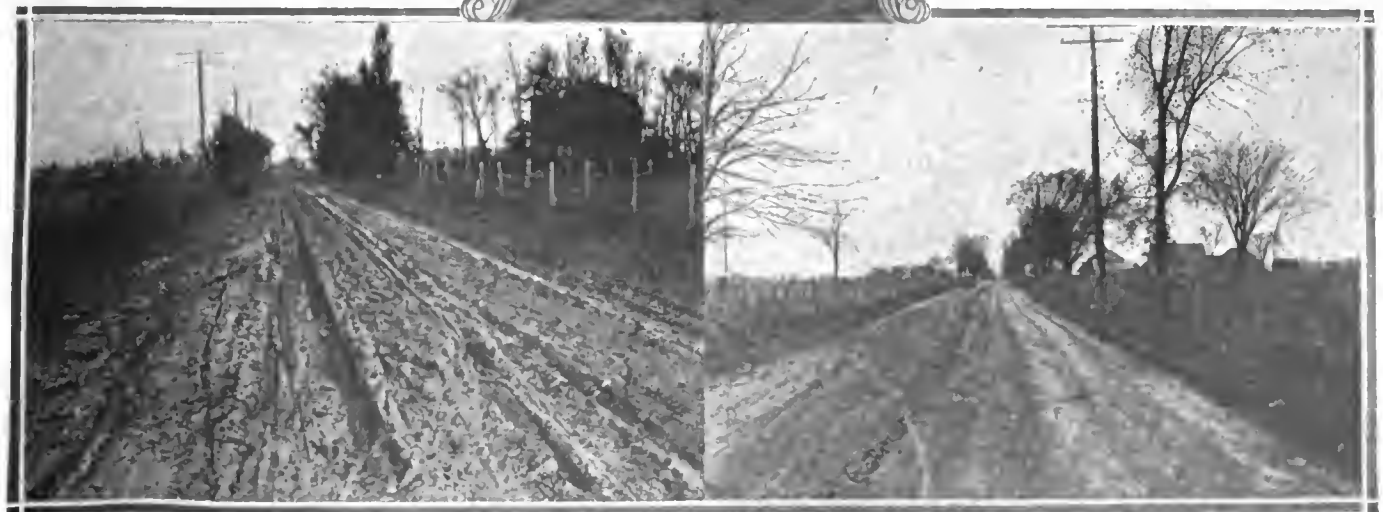
Left: A stretch of road before dragging. This road was covered with a soft clay mud to the depth of about 5 inches
